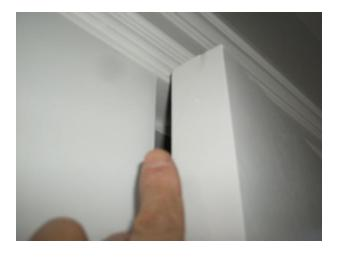
The pocket door to the master closet is rubbing and needs to be adjusted.
