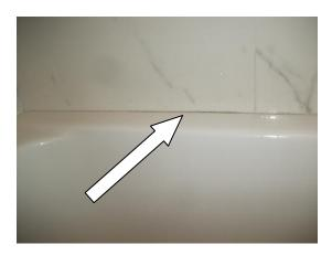
In the garden level bathroom the tub perimeter also needs to be sealed. However you will also need to touch up the grout in the tub corners.
