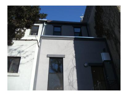
The widows throughout the building have been replaced with new double hung thermo panes. From the outside these windows appear to be properly installed. A generous bead of caulking or sealant was observed at the window perimeters.
