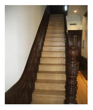
However the newel post on the  $2^{nd}$  floor landing will need to be secured to strengthen the railing to the  $3^{rd}$  floor.
