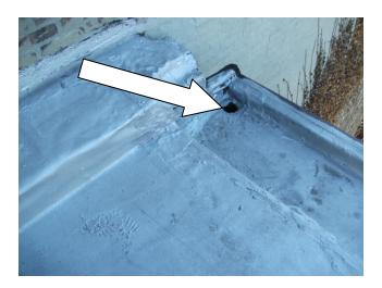
It is hard to forecast how long the existing roof will last. I would recommend re-coating the roof periodically until it is time for a new one Where the roof edge terminates along the common wall with the neighboring building you can see a chip in the sealant. I would recommend having this edge examined and sealed. I would install the proper wall flashing when you install a new roof.
