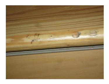
These stairs have been equipped with the required continuous handrails which are original and have been re-finished. Most of these railings proved to be properly secured.
